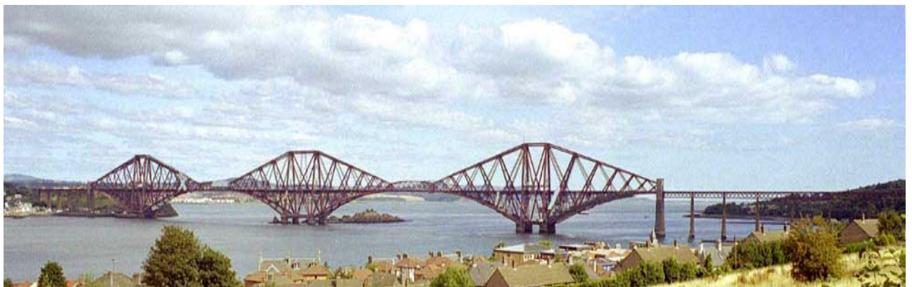
Firth of Forth Railway Bridge 1890, Scotland
